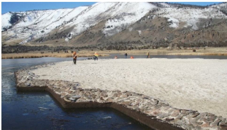
Completing the floating island at Dutchy Lake, Oregon
